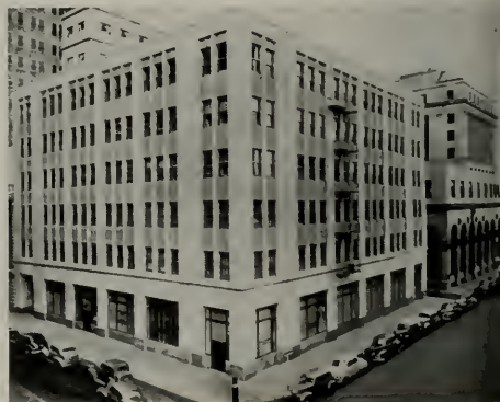
The Cahill Building on California Street near Battery is the latest in modern buildings along the financial section. Many insurance firms and shipping companies are located here including: Pope & Talbot, Inc., and the Marine Exchange.
